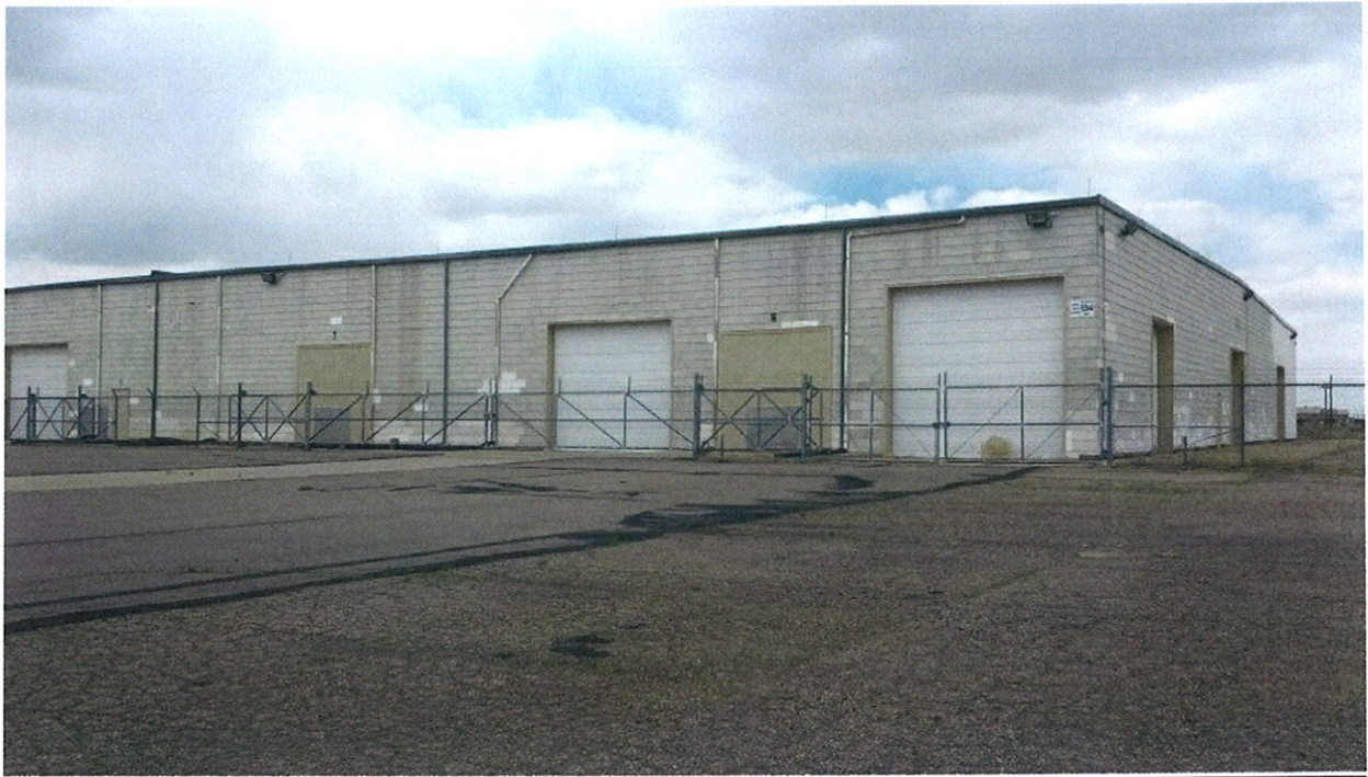
Figure 1 Building 594 East Exterior
